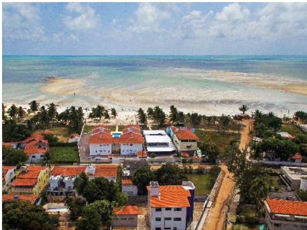
Photo 3 Development and extension of natural sandbars. This has a similar cost and maintenance as beach replenishment.
