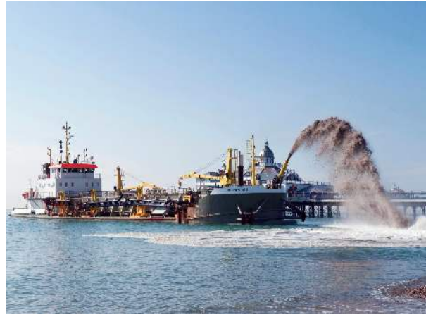
Photo 2 Beach replenishment high maintenance cost and £20 per cubic metre so could be quite expensive.
